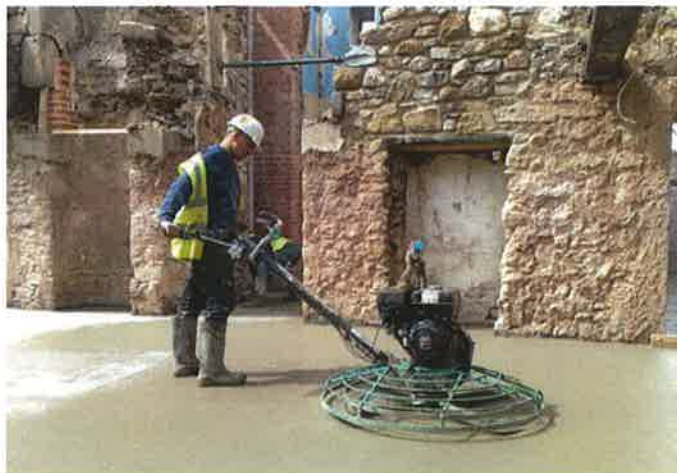
Power float equipment
